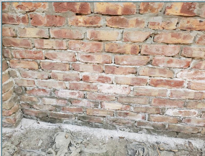
Image: Effects of salinity in coastal areas, areas where houses are exposed to salt water and wind, where salt accumulates and initiates building decay (2023)
