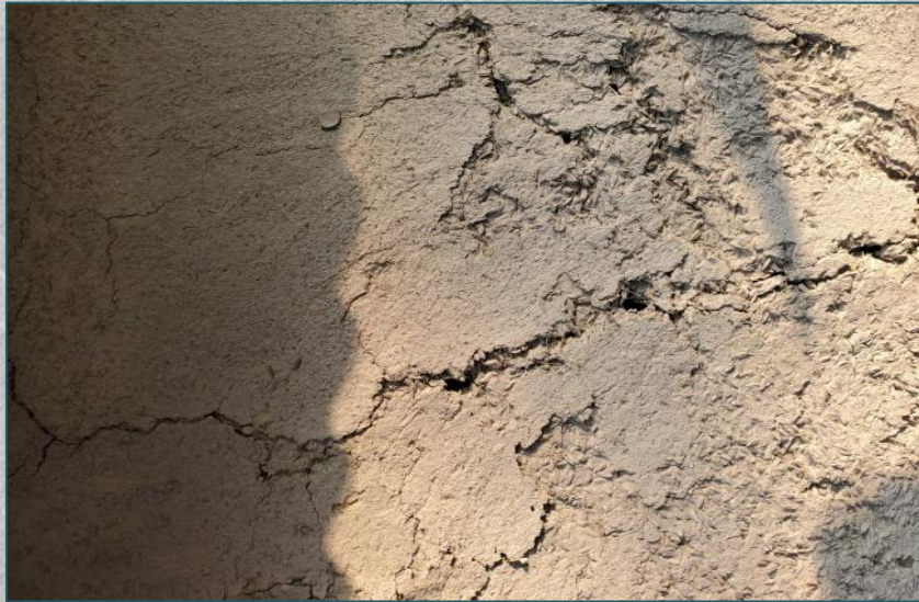
Figure: Damage to wall-coating of mud houses due to salinity in coastal areas (2022)
